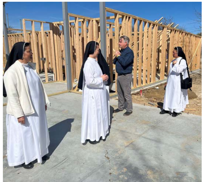
Sisters survey building progress with project architect, Scott Martsolf, AIA
